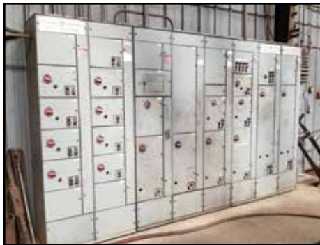
GENERAL ELECTRIC Master Control Center
